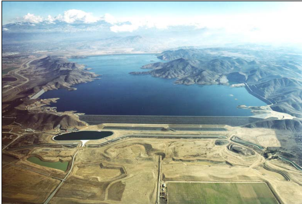
Figure 1. Oblique view of the Diamond Valley Lake.
