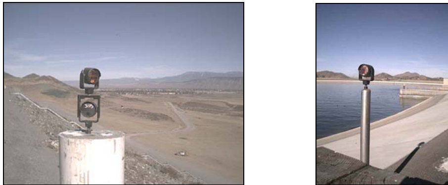
Figure 4. Pillar monuments with the target prisms.
